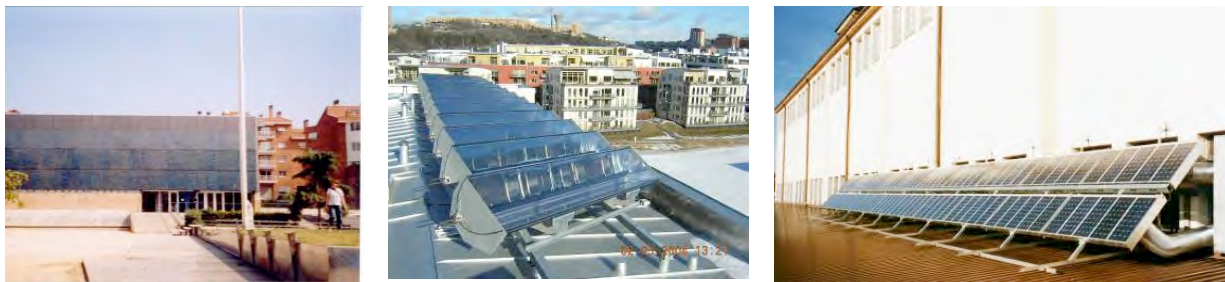
Figure 2. (a) Ventilated PV façade of the Mataro public library in which the heat is recovered and used for space heating and solar cooling, (b) concentrating PV/T system (Vattenfall), (c) PV/T air collector (Grammer KG).
